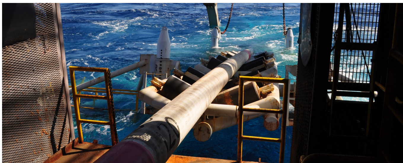
Image: Greater Western Flank Phase 1 pipeline installation in 2014
