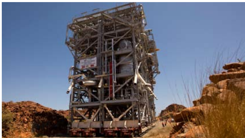
The main liquefaction module travels to site.
